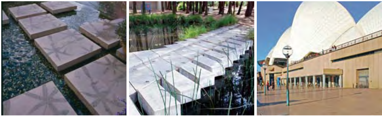
FIGURE 134 Precast paving units allow easier construction over water
