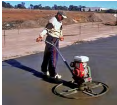
FIGURE 31 Power trowelling concrete surface
