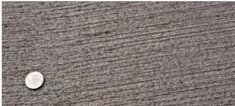
FIGURE 64 Medium to coarse broomed texture suited to industrial applications
