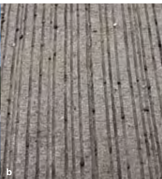
FIGURE 65 Tined finish on roadway – note set pattern in spacing of grooves [a] Tining operation [a] Tined finish
