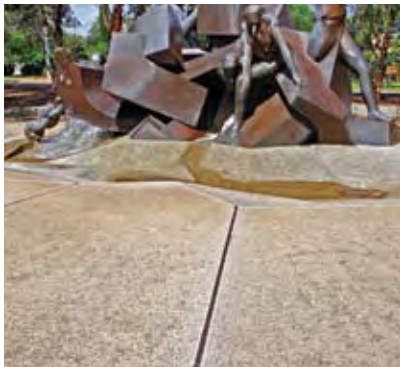
FIGURE 181 Bronze strip, sealed both sides to prevent dirt entry
