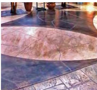
FIGURE 182 Patterned 10-mm-thick topping designed to conceal cracking in substrate
