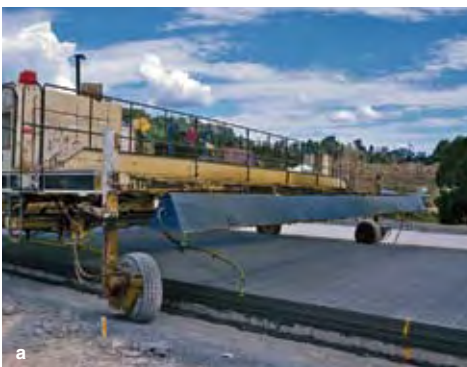
FIGURE 65 Tined finish on roadway – note set pattern in spacing of grooves [a] Tining operation [a] Tined finish
