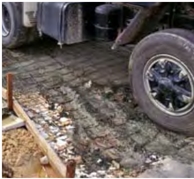
FIGURE 137 Rigid concrete pavements are unable to span over areas of poor subgrade (eg softened by water saturation)
