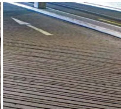
FIGURE 66 Grooves formed in steep ramps for drainage
