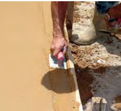
FIGURE 30 Hand floating edges to match levels, fill hollows, compact concrete and round edges to reduce spalling
