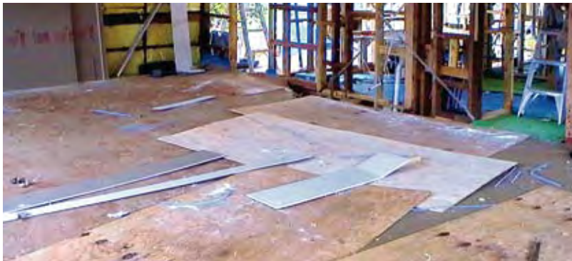
FIGURE 192 Protection of polished concrete floor using felt and plywood sheeting
