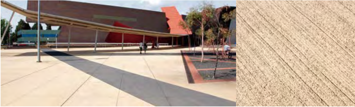
FIGURE 62 Light broom texture can provide a functional and attractive finish
