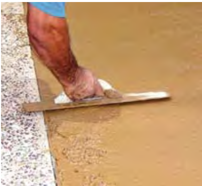
FIGURE 30 Hand floating edges to match levels, fill hollows, compact concrete and round edges to reduce spalling
