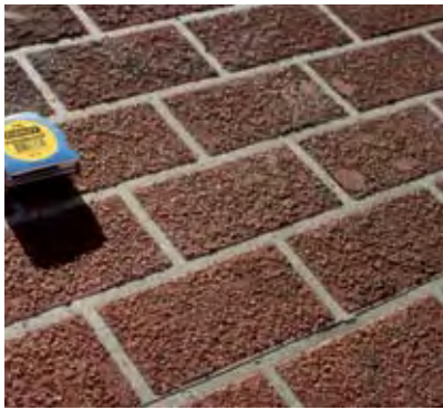
FIGURE 101 Various surface textures can be applied to improve slip/skid resistance
