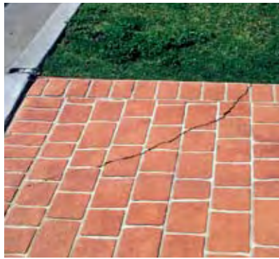
FIGURE 137 Rigid concrete pavements are unable to span over areas of poor subgrade (eg softened by water saturation)
