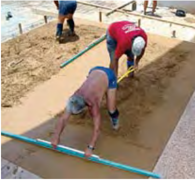
FIGURE 28 Screeding concrete surface to level/profile
