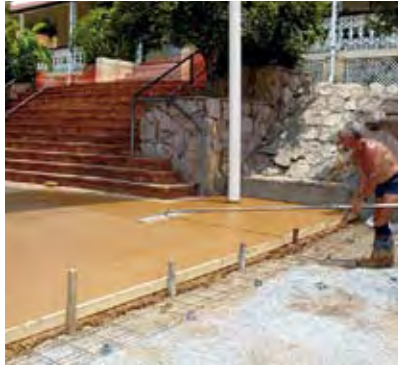
FIGURE 29 Bullfloating concrete surface
