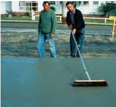
FIGURE 63 Broomed finish to provide slip and skid resistance
